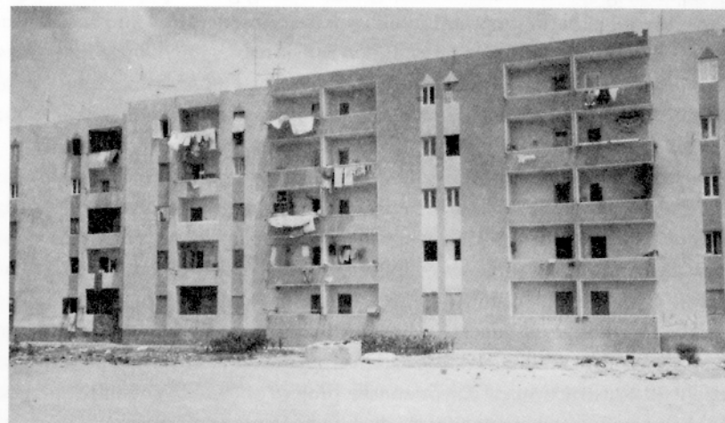
Tenth of Ramadan apartment block (photograph by Omnia El Shakry, July 1996).
